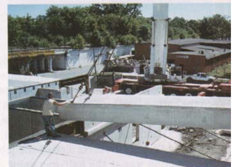
Braced garage walls await double-T roof elements.
