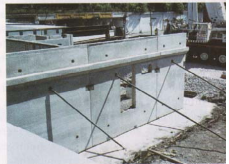
Braced garage walls await double-T roof elements.
