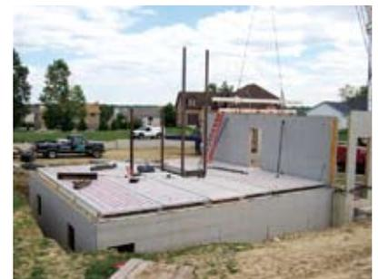
*The speed with which precast concrete wall panels and flooring panels can be erected can be seen in the Aurora, Ill., home, where only a few components are needed to erect the entire shell of the home.*
