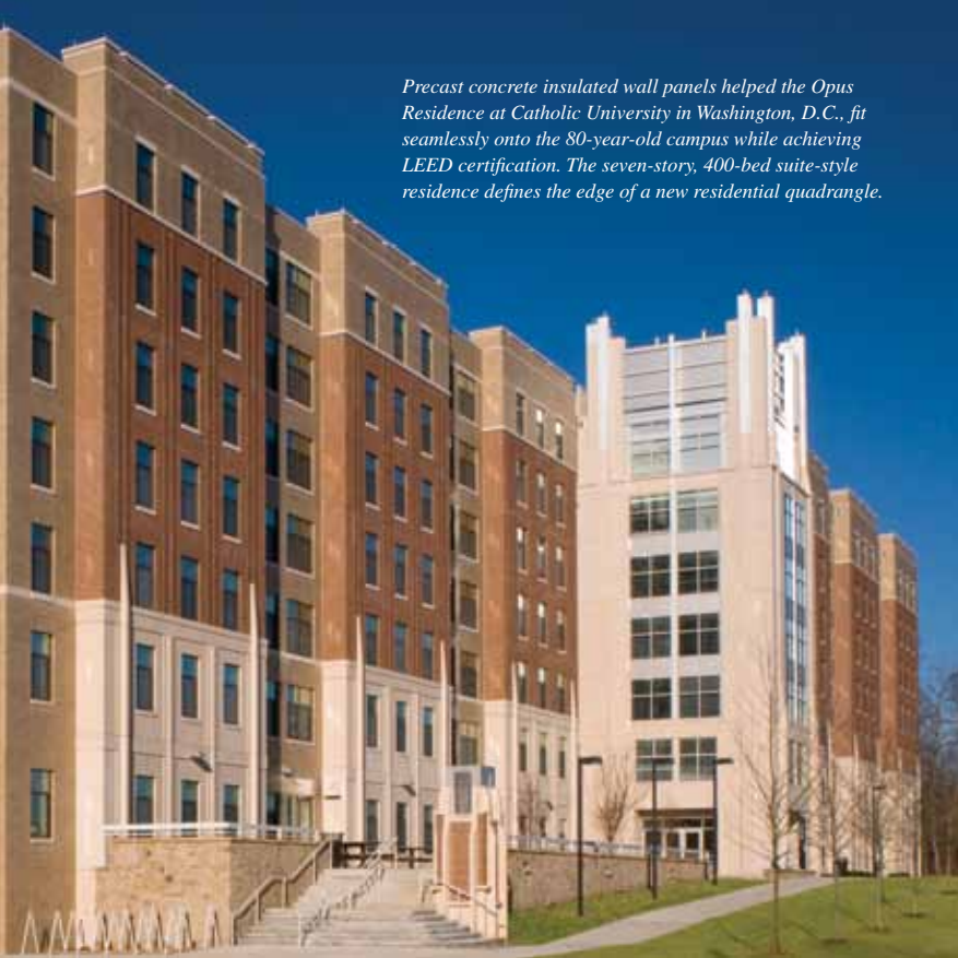
The large size of the panels minimized the number of joints, while casting 3-foot return legs with thin brick on both sides of the punched window units provided a traditional running-bond appearance.
