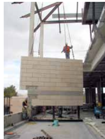
Panels were cast without full-sized stones joint overlaps to avoid creating noticeable vertical joints. Once the panels were erected, crews handset the missing stones to cover the joints.
