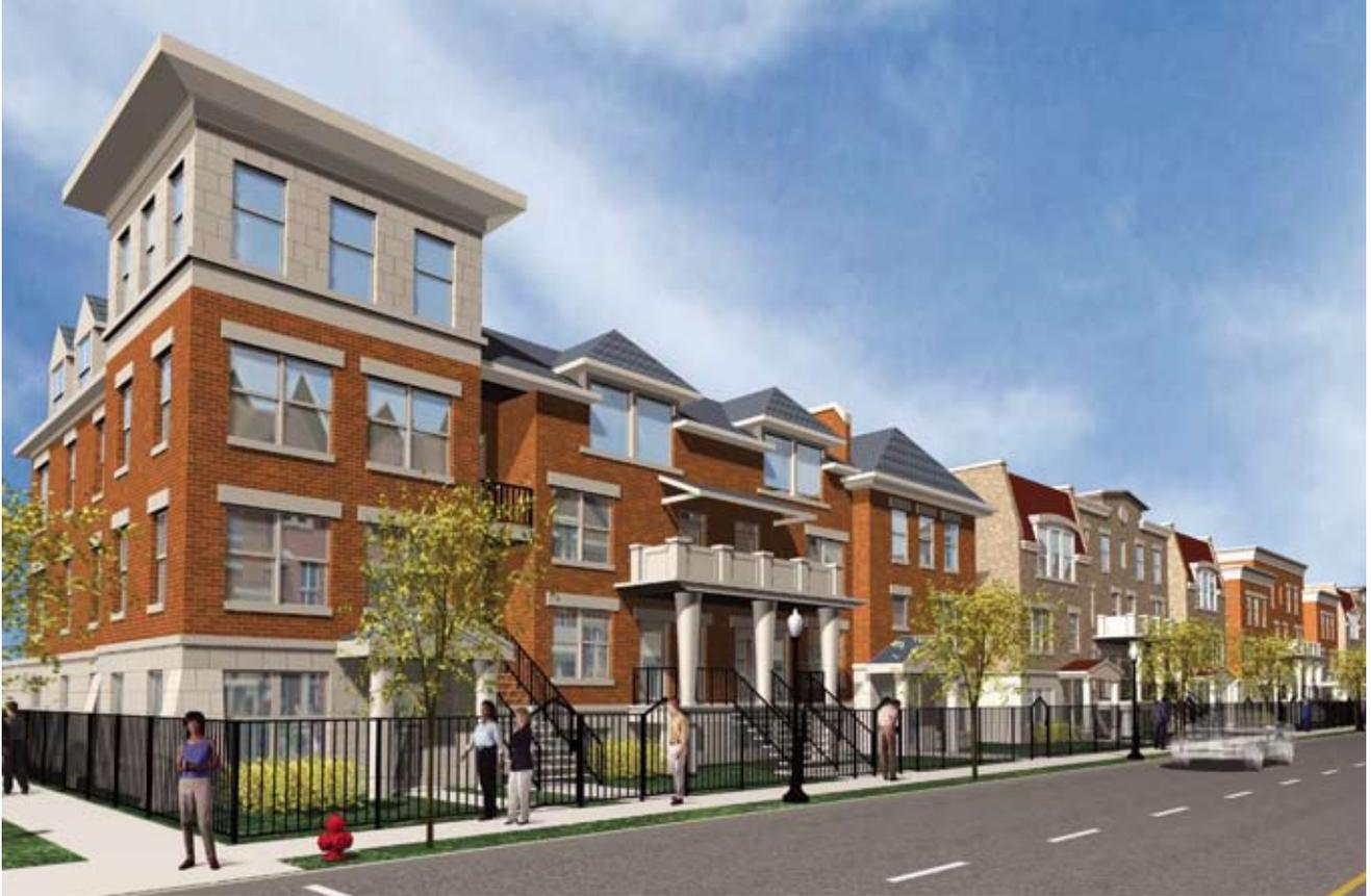
*Piekarz Associates Architects in Chicago has been designing single- and multifamily housing for many years using precast concrete panels. The latest designs feature two finishes: embedded thin brick on top with a rusticated-stone appearance below.*
