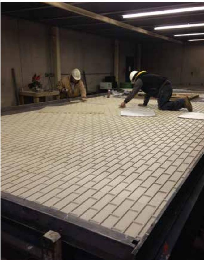
Following the layouts on the architectural and engineering drawings that are specific to every panel, workers place the plastic formliner on the rotating steel tables prior to concrete placement.
