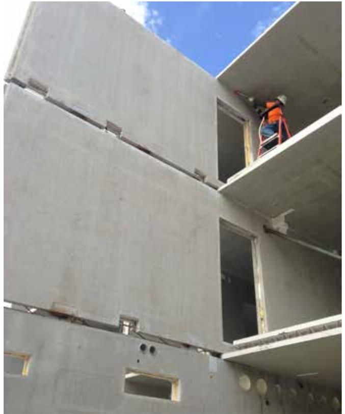
The fully insulated wall and floor panels were erected in a multi-phase operation, allowing timely access to be scheduled for other trades.
