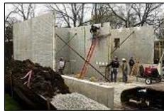
The Red Cross, with about 30 other organizations and the City of Aurora, is building the first fortified home in Aurora on Benton Street. A fortified house is made of pre-cast concrete and designed to stand up to tornadoes, hurricanes and hailstorms.
